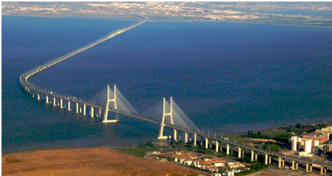
Figure 3.1 : Vasco da Gama bridge 7
