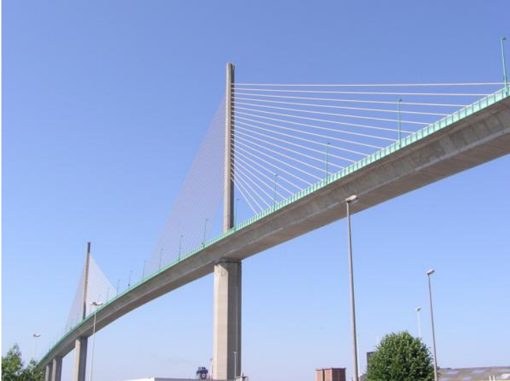
Figure 1.2 : Brotonne bridge, 320m span (1977) 2
