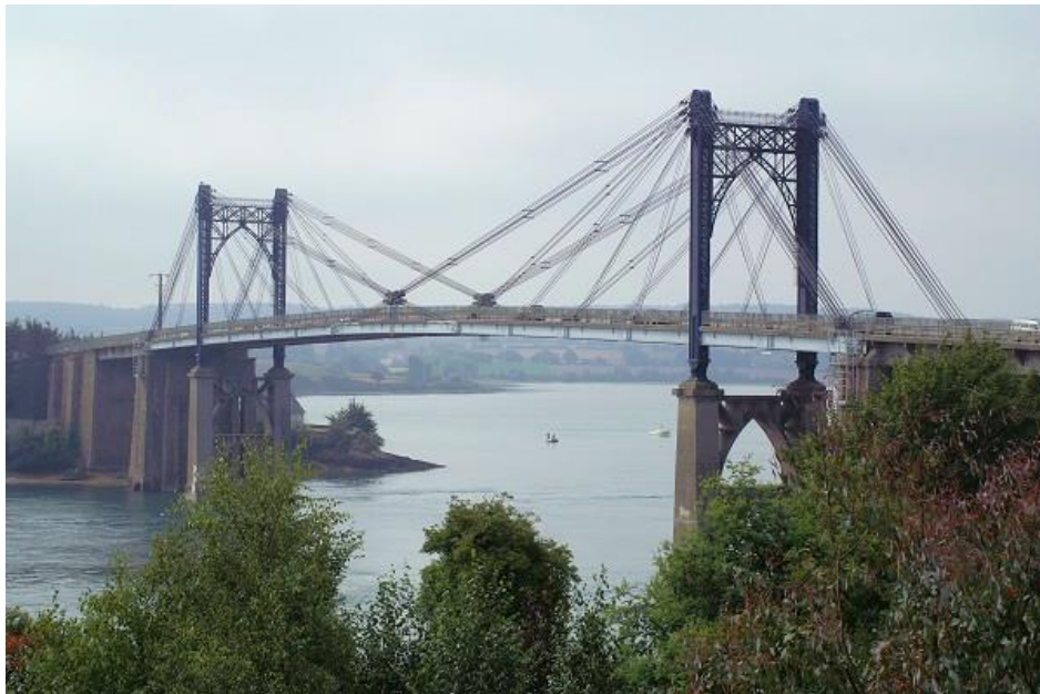
Figure 1.1 : The Lézardrieux bridge, 112m span (1925) 1
