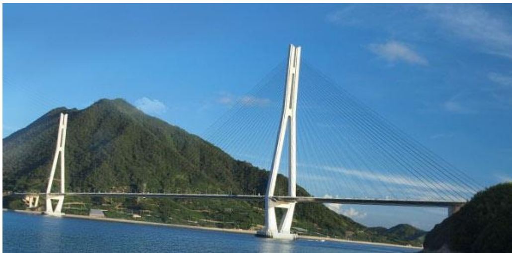
Figure 1.5 : Tataru bridge, 890m of span (1999) 5
