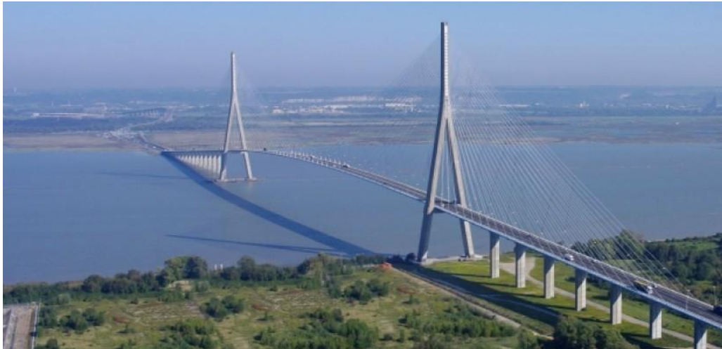
Figure 1.4 : Normandie bridge, 856m span (1988) 4
